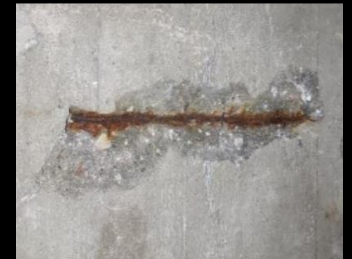
Spalling with corroded rebars (Spalling + Rust)
