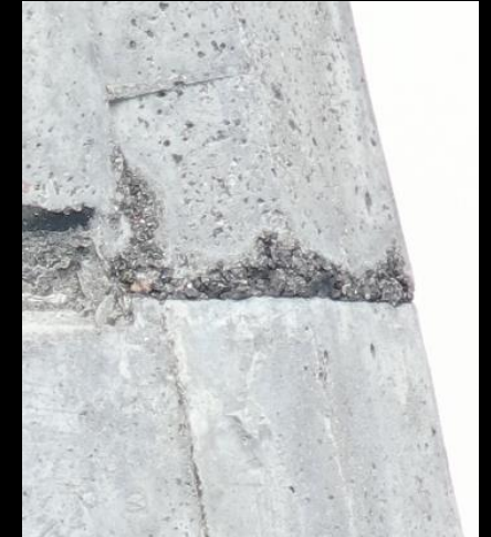
Spalling/ casting defects with visible aggregates
