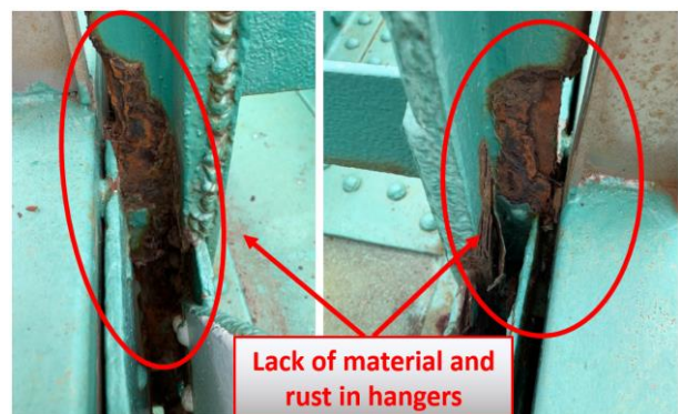
Figure 2. Example of damaged hangers.
